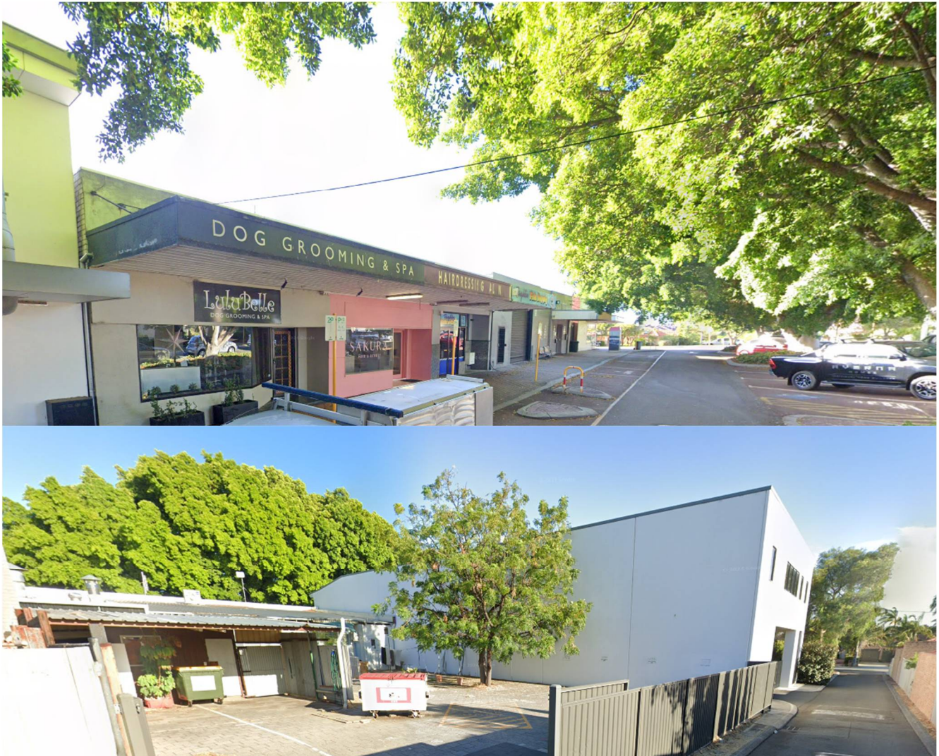
Figure 3 -The existing development on the subject land. The top photo is along the land's Muriel Avenue frontage and the bottom photo is from the Azurite Lane.
