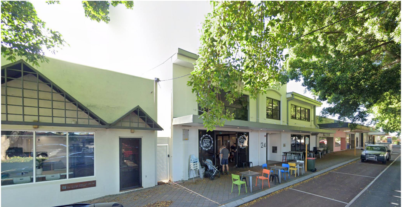
Figure 4 – Examples of existing developments within the Muriel Avenue commercial strip. The current development on the subject and comprises a poor built form character and represents under development of land within an established local centre.
