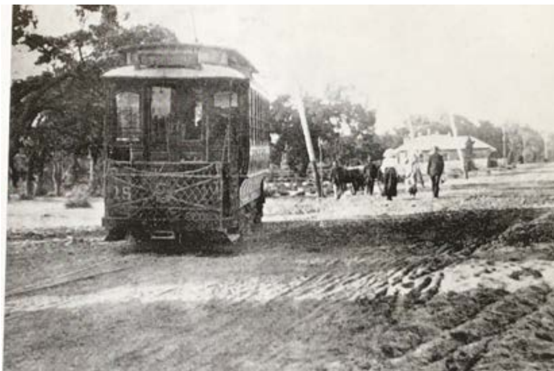
Tram 15 moves through the points onto the siding at the Osborne Park terminus. n.d.
