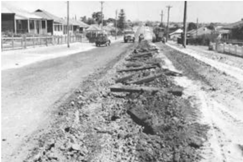
Tramlines being taken up along Main Street.
