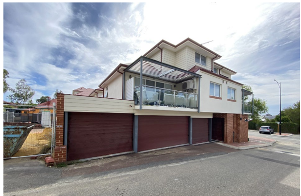
Figure 8 Rear view of 760 Beaufort Street
