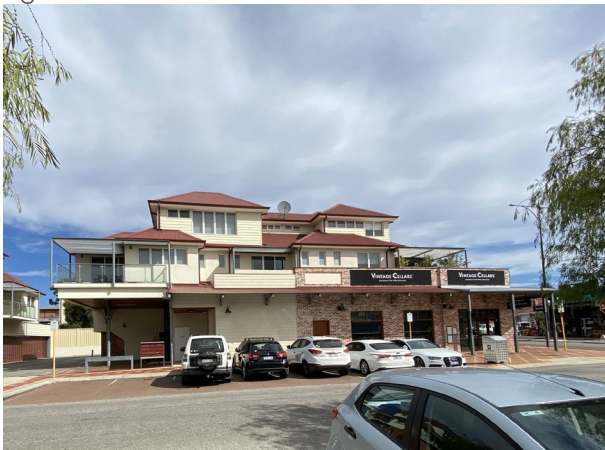
Figure 9 Side view of 760 Beaufort Street
