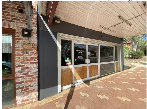
Figure 6 Main shopfront of existing building
