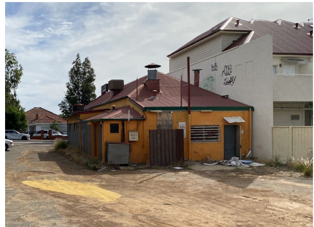
Figure 4 Southeast view of existing building
