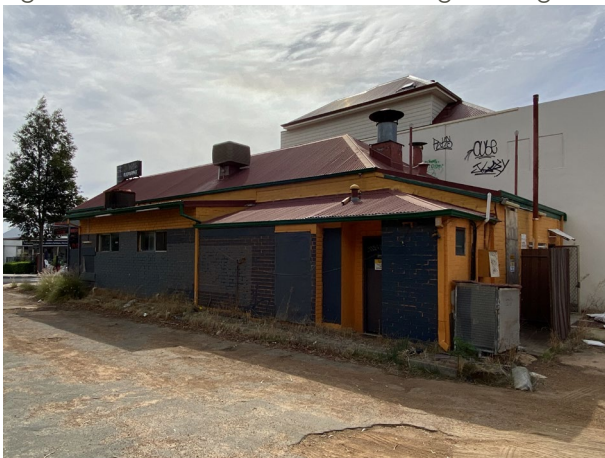
Figure 5 Western view of existing building
