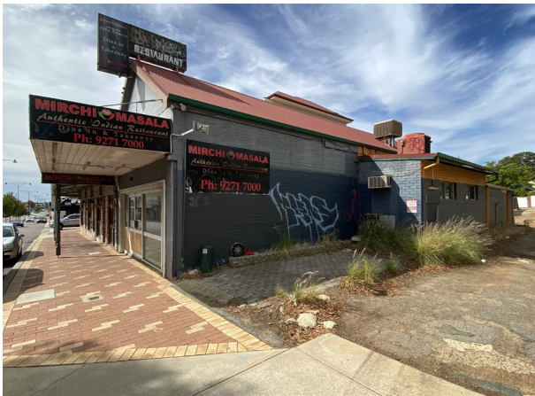
Figure 3 Northwest view of existing building
