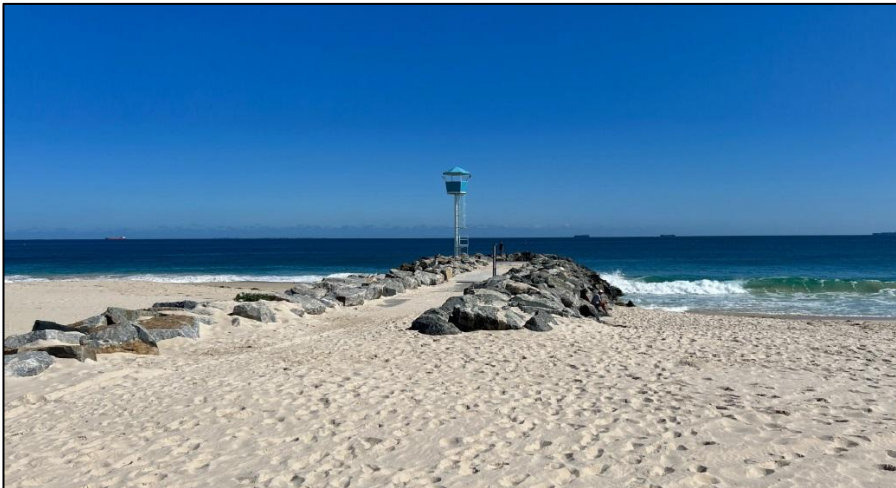
Figure 3 – Groyne at City Beach
