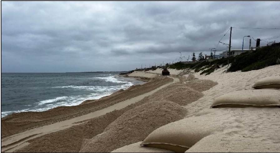
Figure 1 – Sand Nourishment at Mettams Pool
