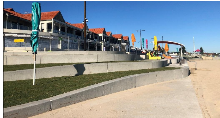
Figure 2 – Seawall at Rockingham
