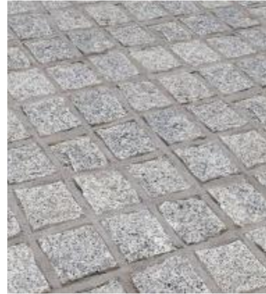
GRANITE SETT FEATURE PAVING
