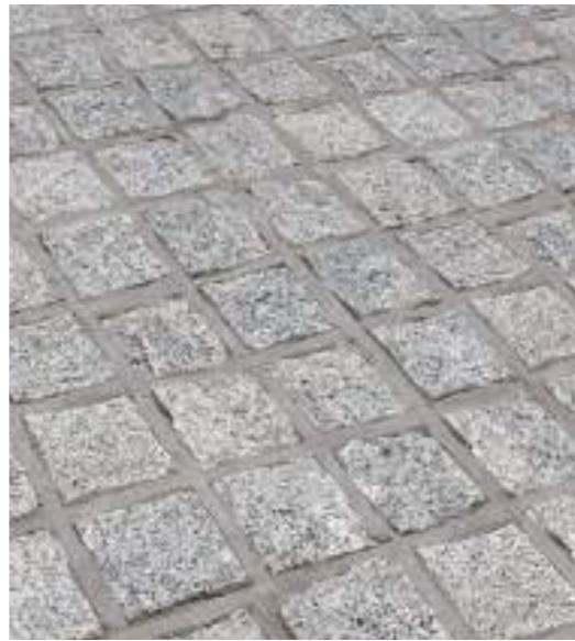
GRANITE SETT FEATURE PAVING
