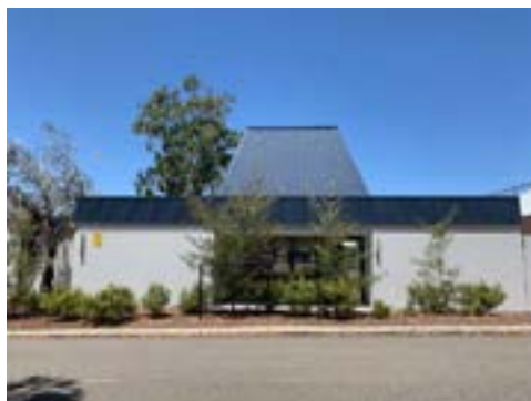
Dianella Library, following the 2014 refurbishment ( element , 2019)
