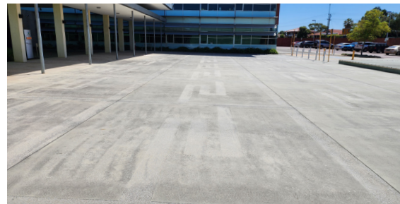
04 View of forecourt showing its gradient fall towards Cedric Street + concrete patterning
