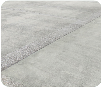
Existing sandblasted green concrete
