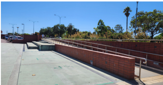
03 Ramp connecting forecourt to Cedric Street
