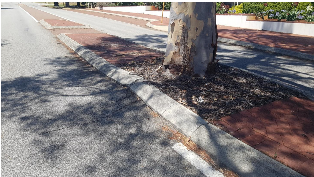
Photo 5: Kerb damage and cracking of the road caused by the roots on Banksia Street, Tuart Hill.
