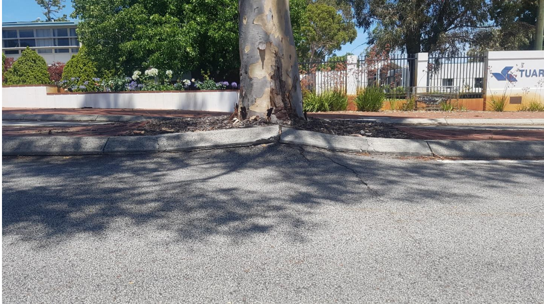
Photo 6: The growing roots have caused significant upheaval of the road surface.
