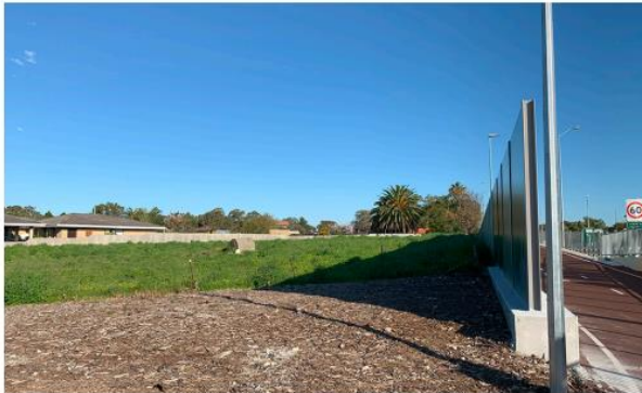
NORTH-WEST CORNER OF SITE
