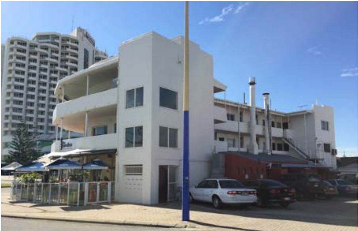
IMAGE 11. SUBJECT PLACE WESTERN AND SOUTHERN ELEVATIONS (2015)
