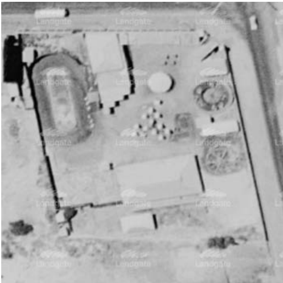
IMAGE 3. HISTORIC AERIAL PHOTOGRAPH OF LUNA PARK, 1965, LANDGATE (RETRIEVED 2015)
