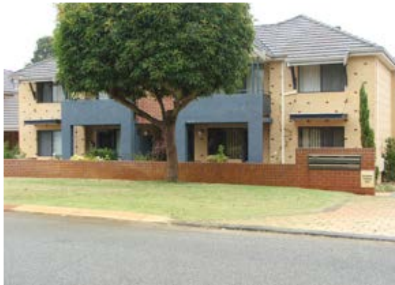
Plate 6 Innaloo R40 – Two storey multiple dwellings
