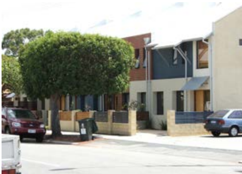
Plate 7 Inglewood, R40 – contemporary two storey multiple dwellings
