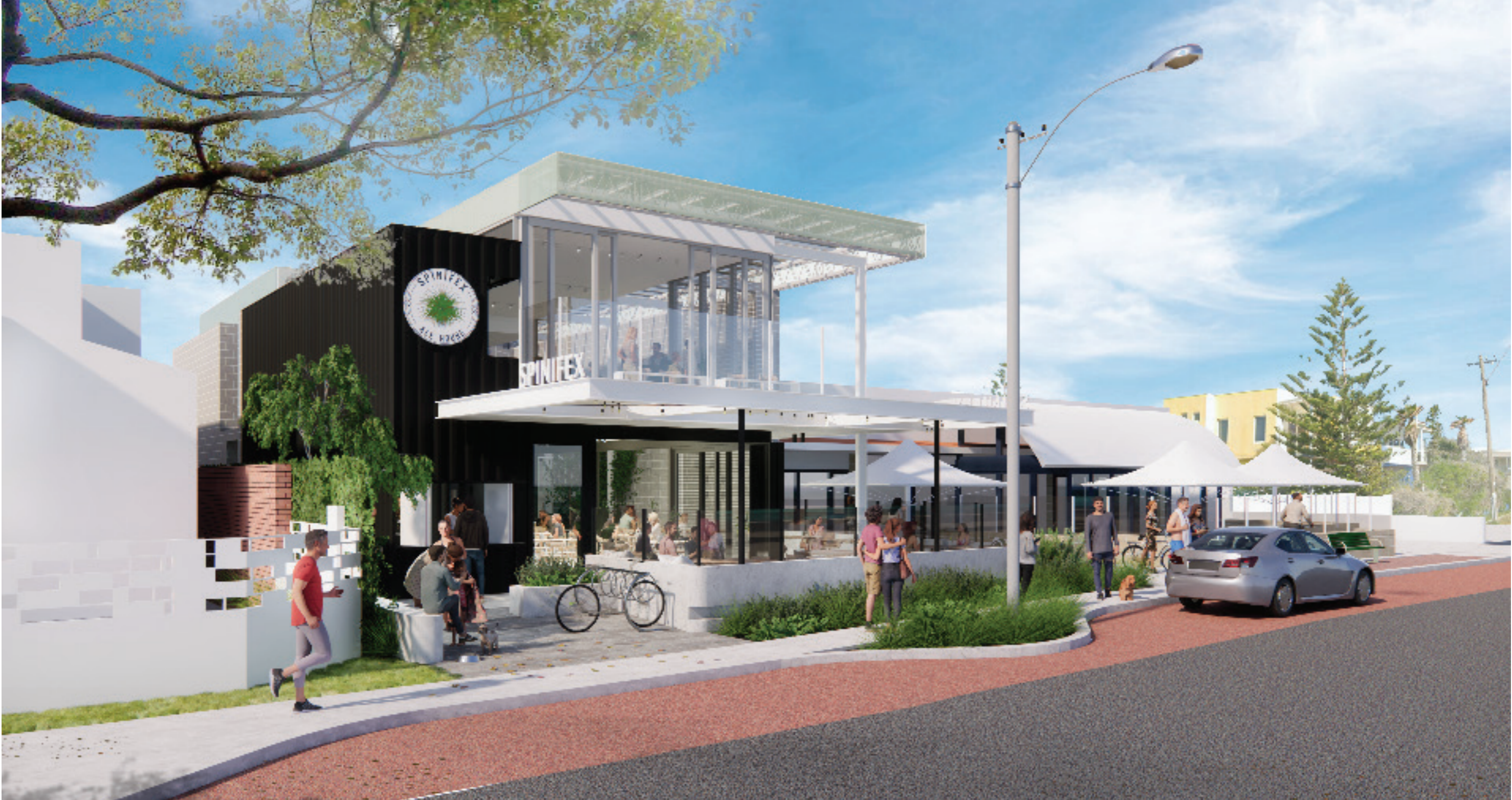
WEST COAST DRIVE - STREET FRONTAGE_NORTHERN APPROACH
