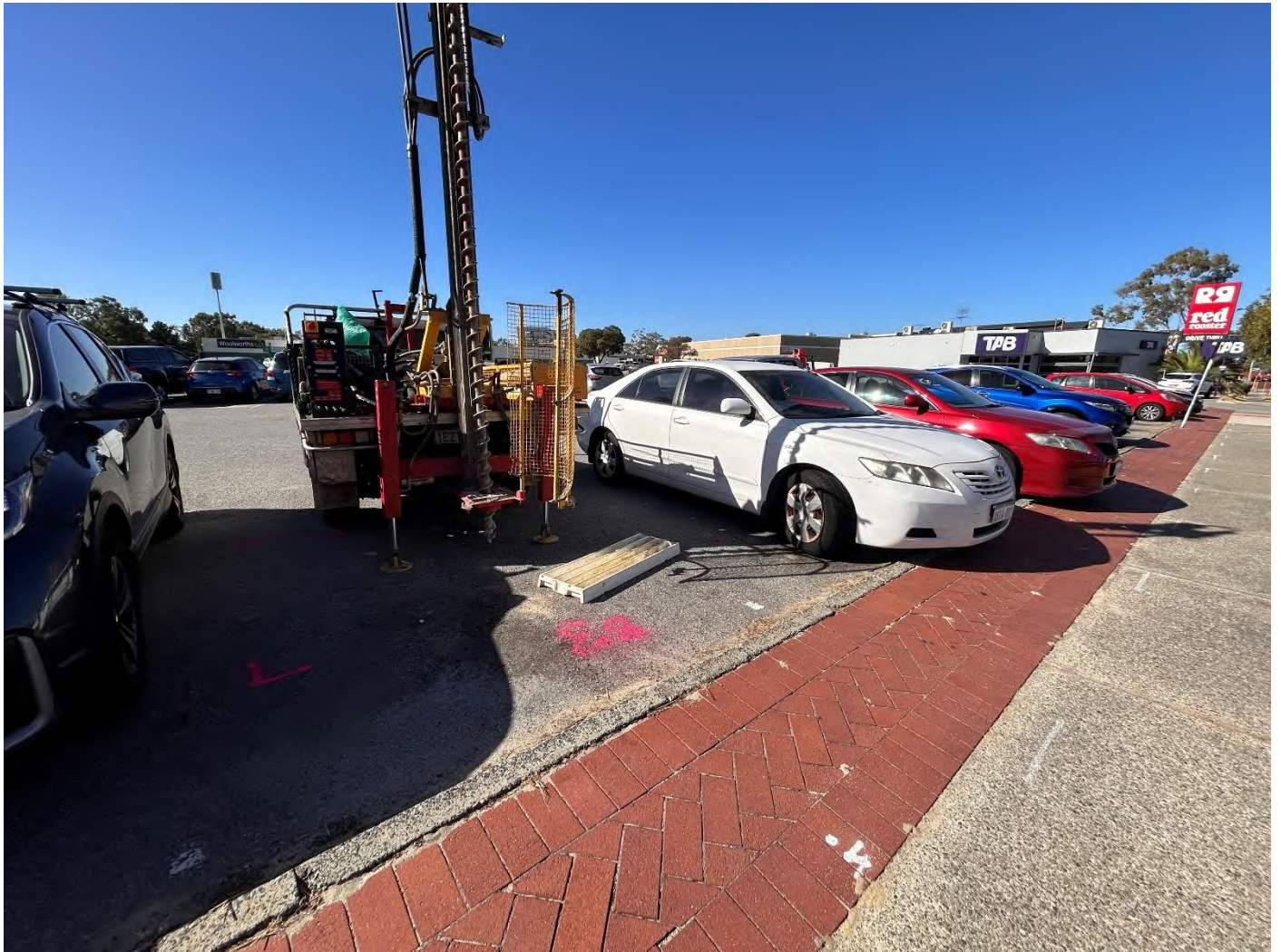
Photograph 6: Facing southeast at BH03 location.
