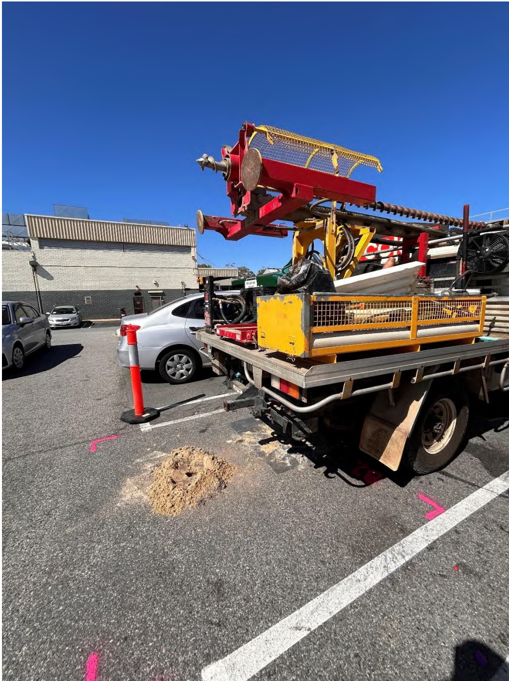
Photograph 4: Facing southeast at BH02 location.
