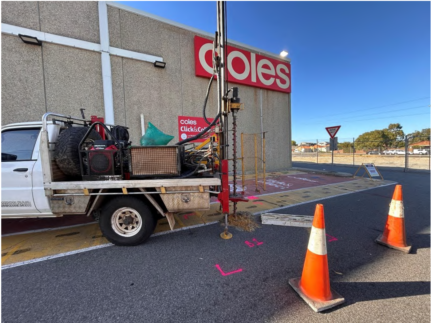
Photograph 2: Facing southeast at BH01 location.
