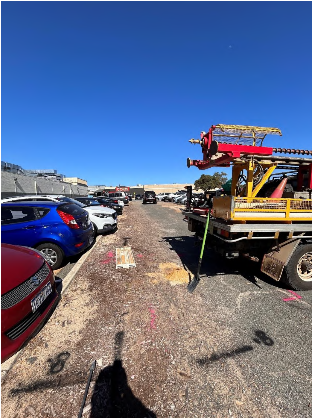
Photograph 7: Facing southwest at BH05 location.
