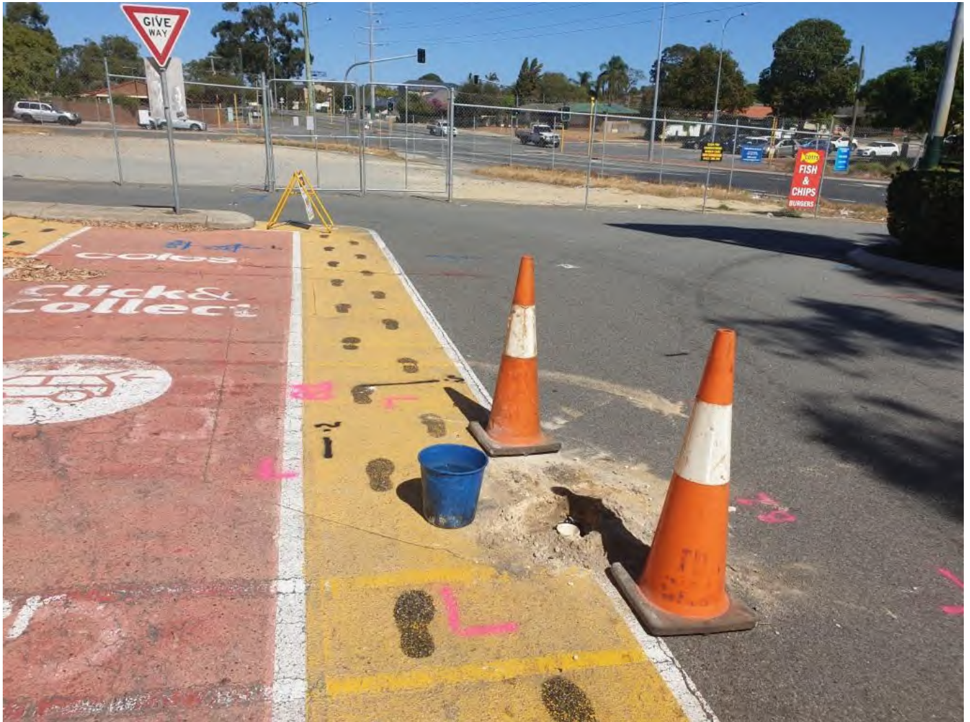
Photograph 3: Facing southwest at BH01 location. IT01 in progress.
