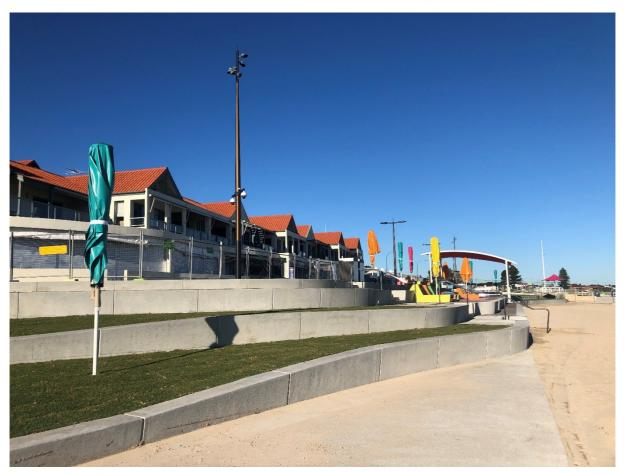
Figure 7.3 Vertical Seawall (Terraced – Rockingham)
