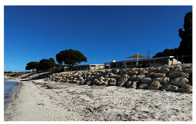
Figure 7.2 Rock Revetment (Rottnest Island)
