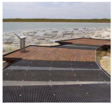
IMAGE 13: FRP WITH MATERIAL CHANGE IN PRIMARY & SECONDARY NODES (ARCHATRAK)
