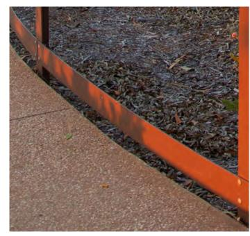
IMAGE 15: CUSTOM KICK RAIL TO WRAP AROUND THE BOARDWALK AND NODES - MINIMUM 300MM WIDE (UDLA)
