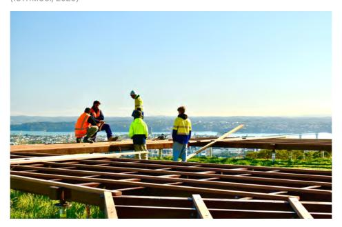
IMAGE 4: CONSTRUCTION WITH SIMPLE SCREW PILES IN MANGAWHAU BOARDWALK (ARCHI PRO)
