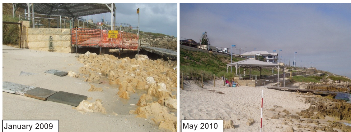
Figure 2.3 Previous Undercutting of Infrastructure at Mettams Pool
