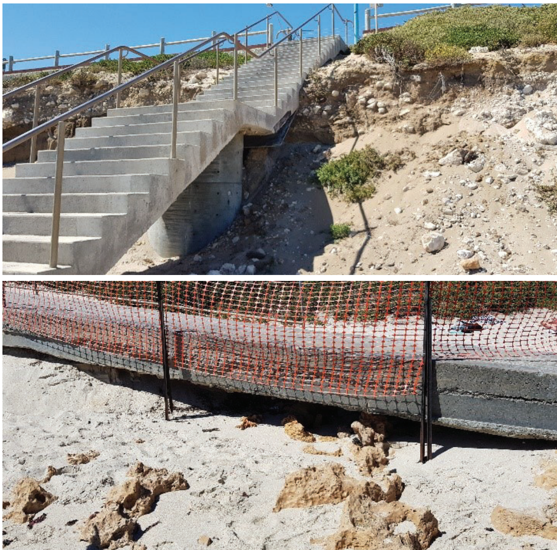
Figure 2.2 Undercutting of Assets at Mettams Pool
