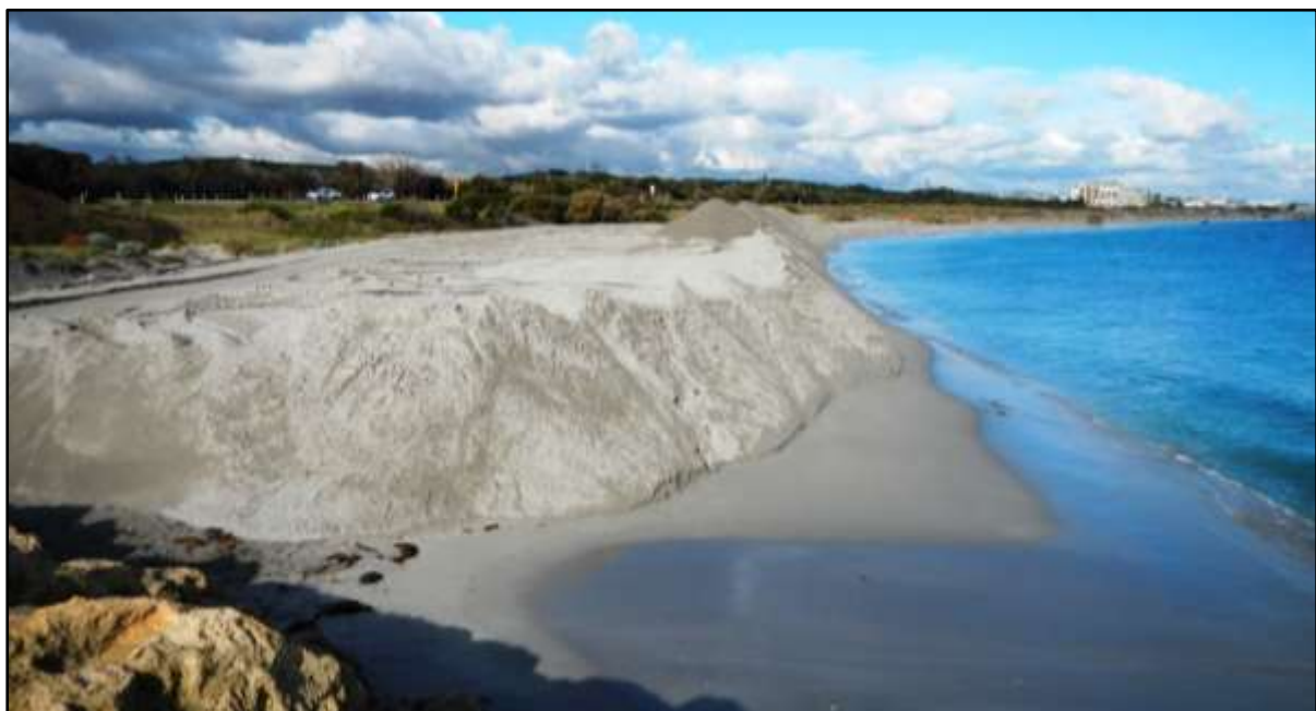
Figure 4-2 Beach renourishment occurring to protect assets at C Y O'Connor Beach, North Coogee
