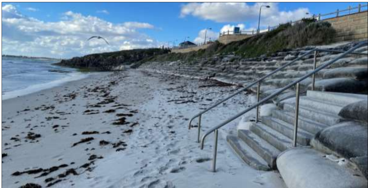
Figure 4-5 GSC seawall at Watermans Bay Beach
