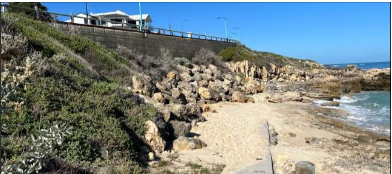
Figure 3-8 Rock protection and retaining wall between Lynn and Bailey Streets
