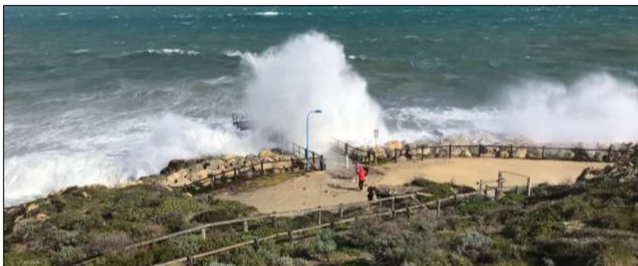
Figure 4-1 Example of wave overtopping of the north beach revetment
