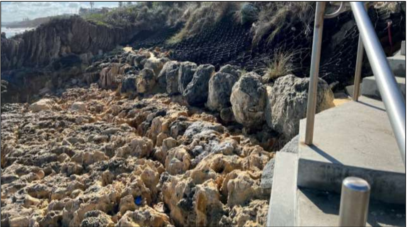
Figure 3-7 Hamersley Pool rock protection and dune retention/restoration (Geocells)
