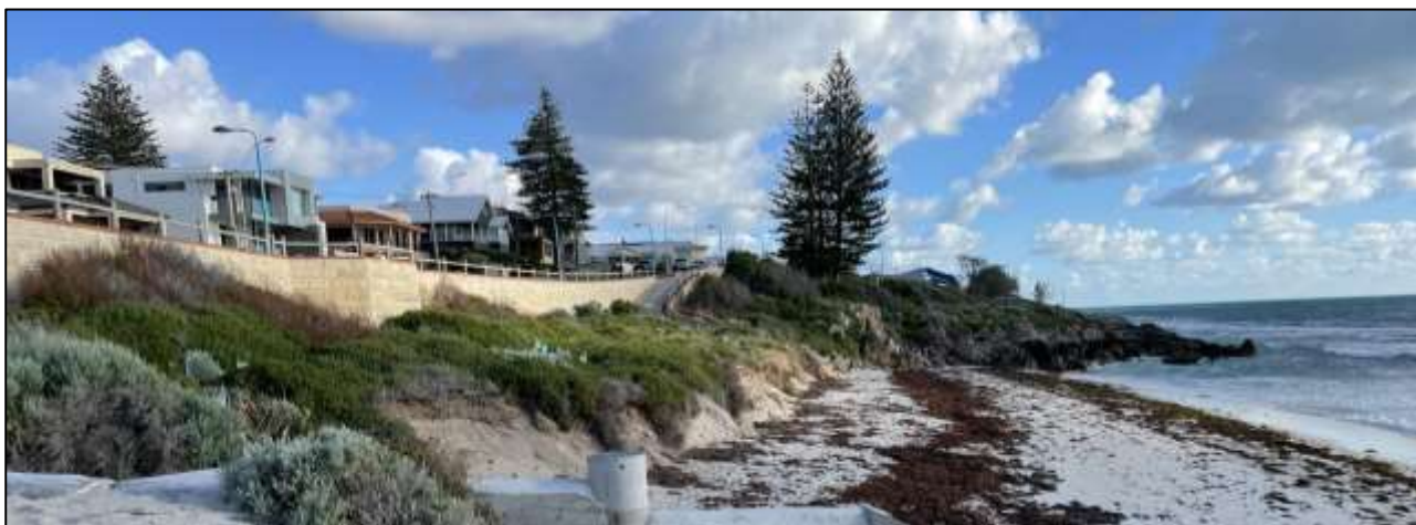
Figure 3-10 Retaining wall along a section of West Coast Drive as well as dune revegetation (Watermans Bay).
