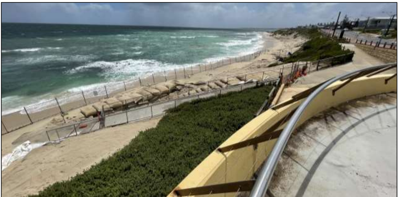
Figure 3-5 Mettams Pool GSC Defence during construction, as well as placed nourishment
