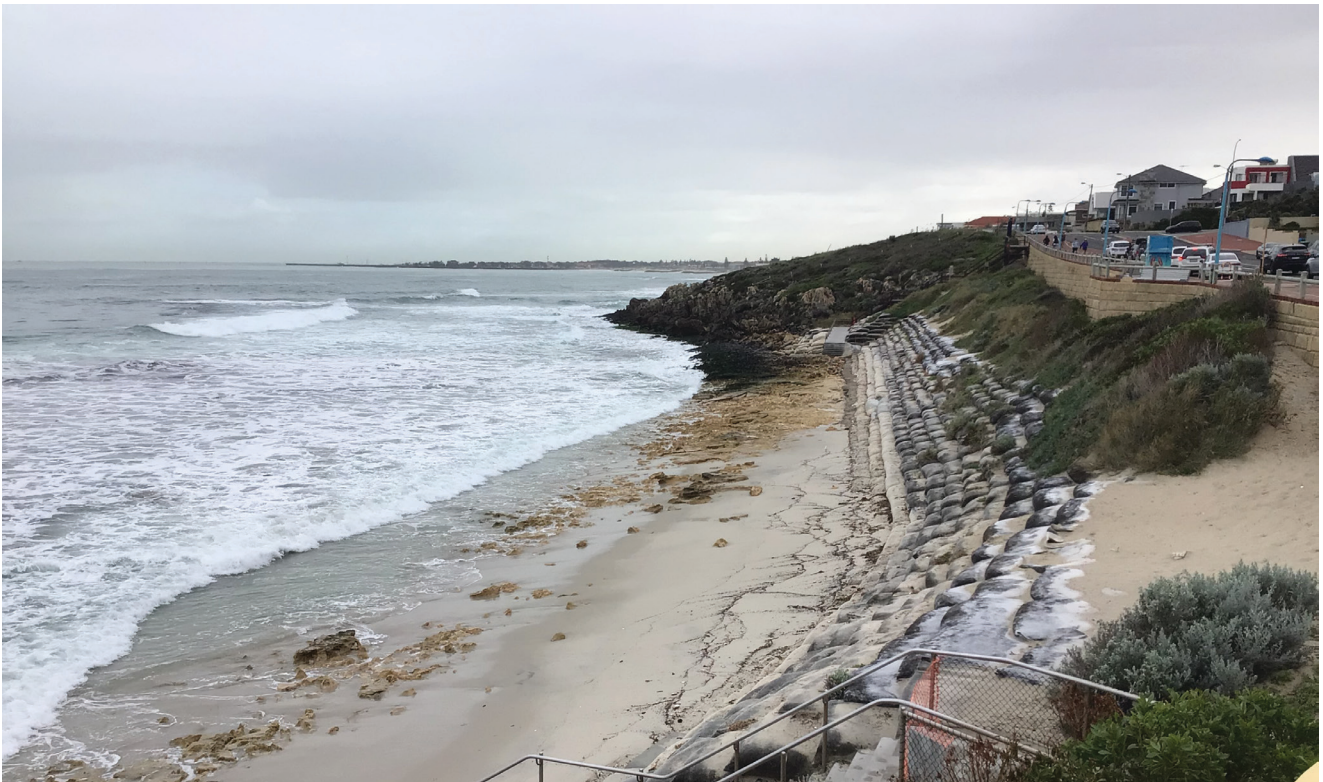
Figure 10: Seawall at Watermans Bay
