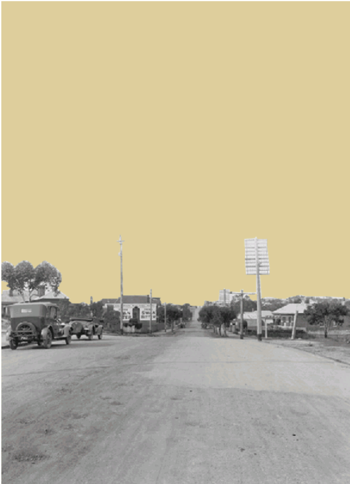
Experimental patch of spramex priming coat method of road. Source: City of Stirling Local History Collection LH000304
