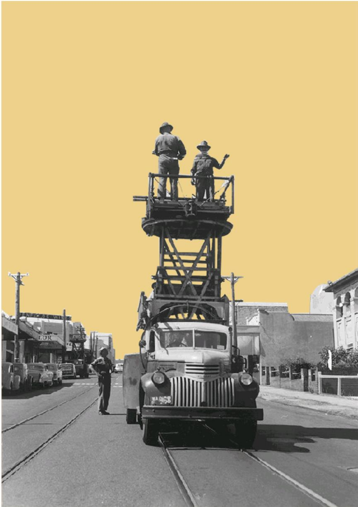
Tram cable maintenance in the Mount Lawley and Inglewood c.1958. Source: City of Stirling Local History Collection LH000139
