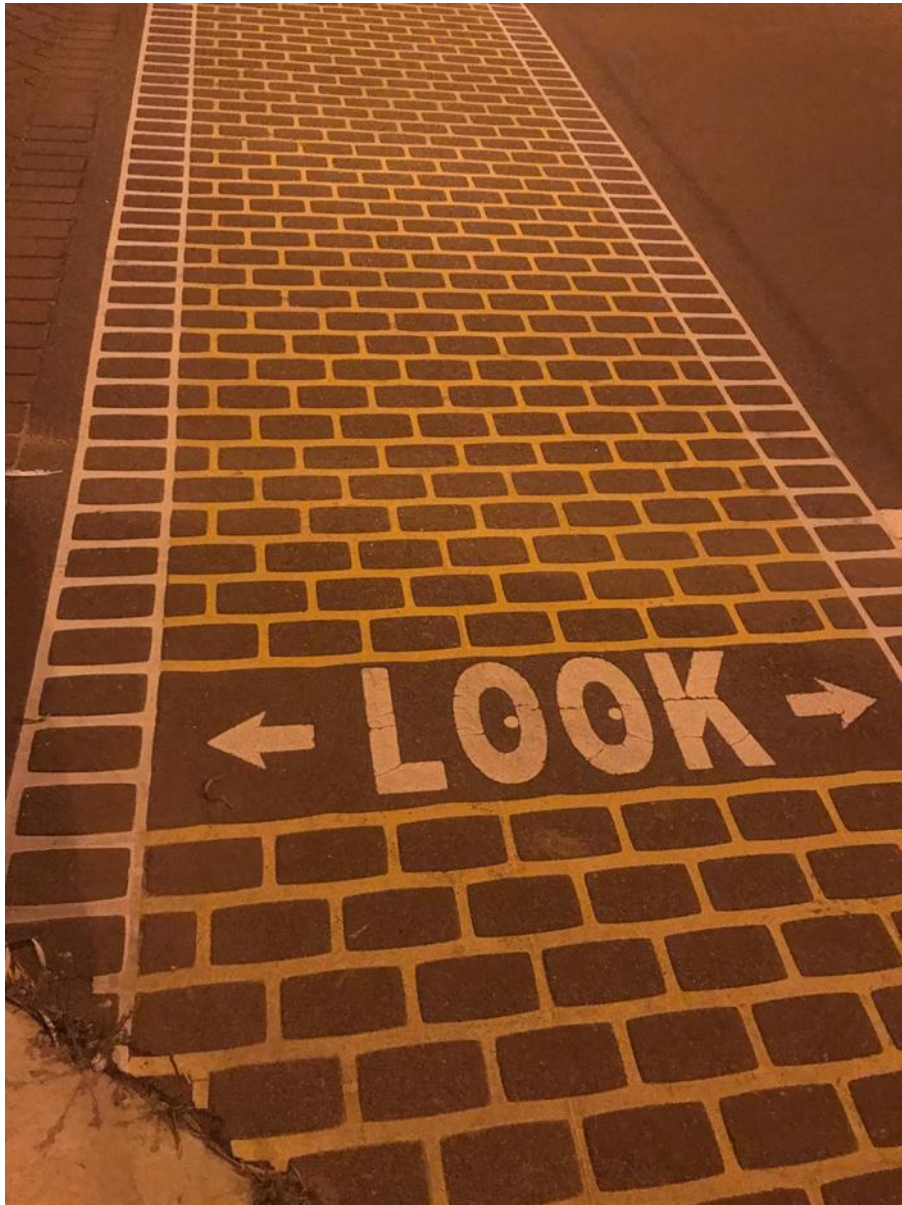
Figure 1 – DuroTherm used at a pedestrian crossing at the intersection of Powell Street and Tyler Street in Tuart Hill
