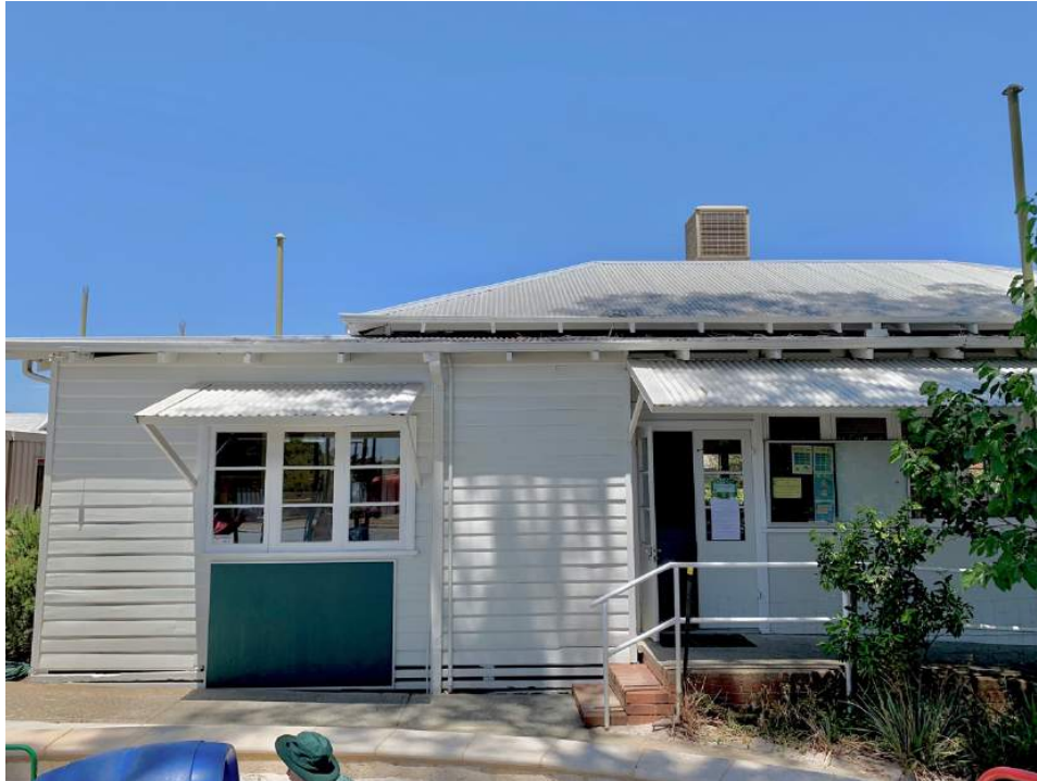
Front elevation of the former Mount Ingle Tennis Club Pavilion (element, 2019)
