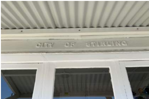
View of signage to the front elevation (element, 2019)
