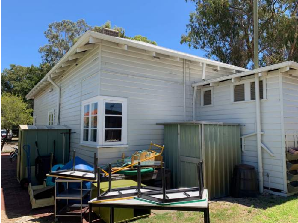
Side and rear elevation of the Former Mt Ingle Tennis Club pavillion (element, 2019)
