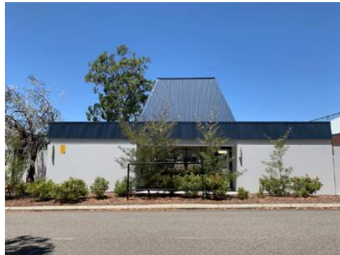
Dianella Library, following the 2014 refurbishment (element, 2019)
