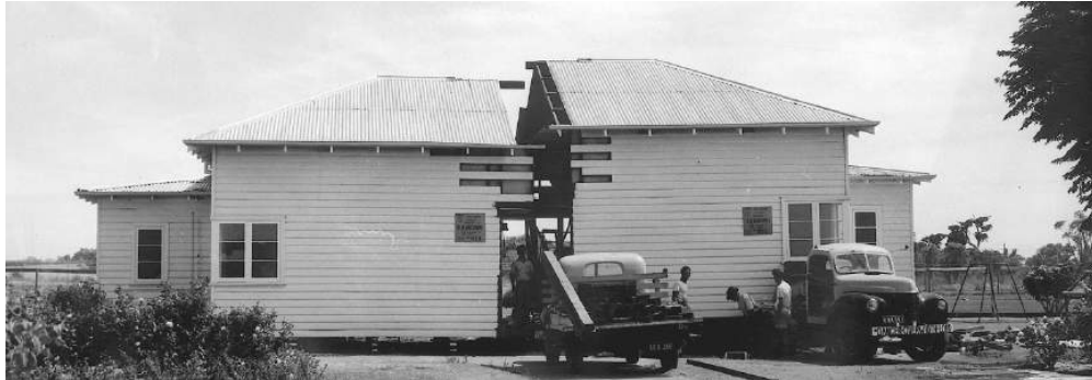
Archival photo of Mt Ingle Tennis Club pavillion being deconstructed for relocation in 1958 (City of Stirling, LH000021)
