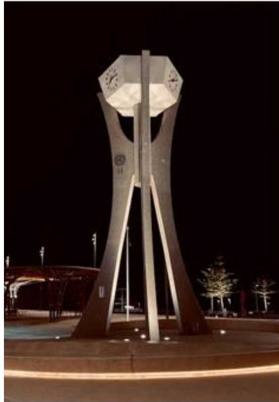
Figure 1: existing white lighting
