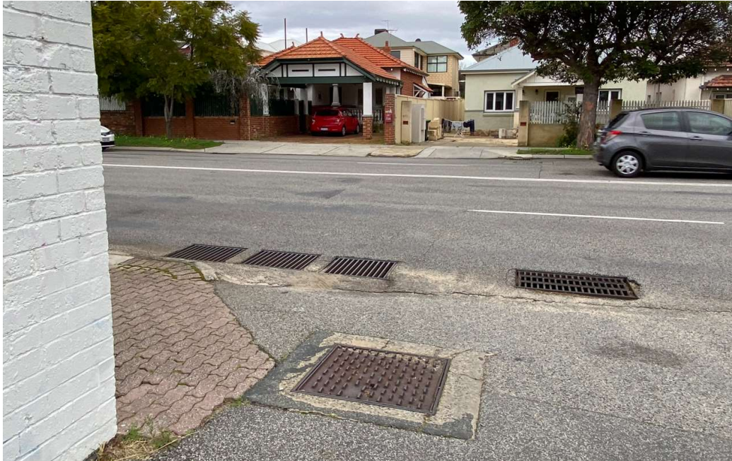
Finding 2.5 – Obscured sight lines between vehicles exiting Klem Lane and pedestrians due to adjacent building
